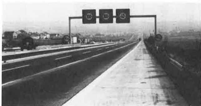
FIGURE 2 Alignment of Elzer Mountain, downgrade direction.
