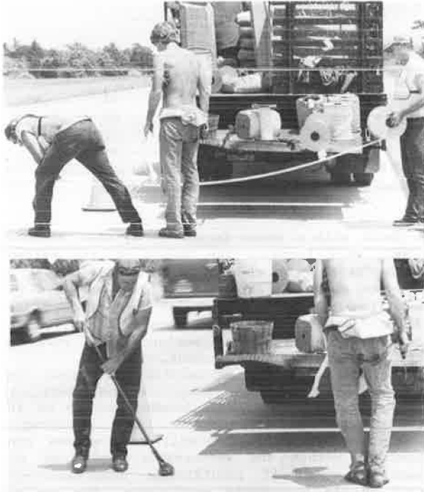
FIGURE 9 Placing stitched cotton piping cord.
