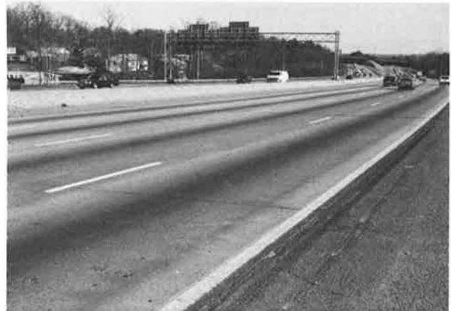
FIGURE 5 Capitol Beltway (I-495), middle section constructed with Prince George's coarse aggregate.
