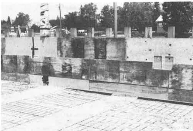
FIGURE 3 Steel bar-mats behind wood faced MSE.
