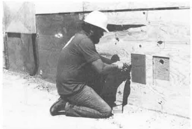
FIGURE 4 Field installation of soil pressure cells behind plywood face.
