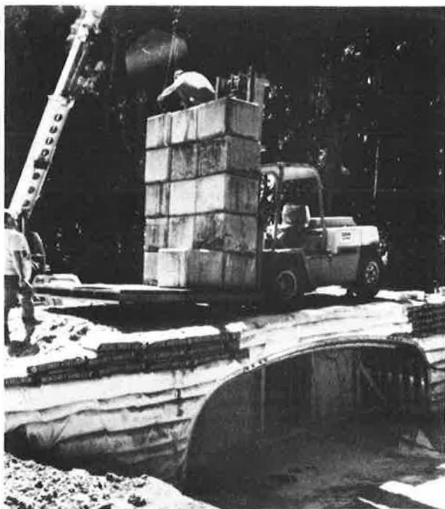
FIGURE 4 Field loading, view from northeast corner of structure.
