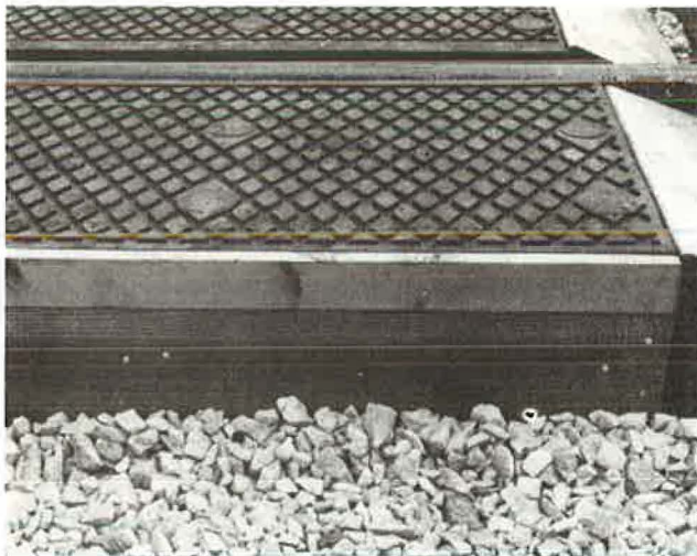
FIGURE 10 The top of a header board can also be designed to facilitate the construction of a flexible sealed joint between the pavement and the crossing.
