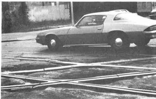
FIGURE 1 A high-type crossing surface is desirable for a rough and dangerous crossing such as this.
