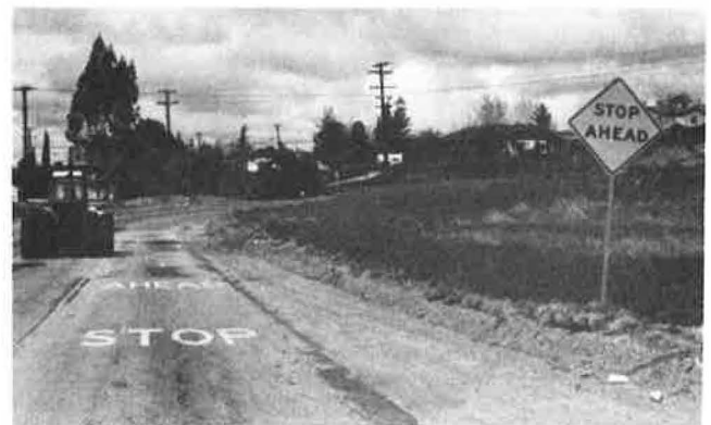
FIGURE 4 Pavement markings and STOP AHEAD sign used to emphasize presence of remaining stop sign after conversions (San Bernardino County, California).
