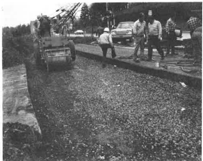
FIGURE 8 A properly designed and installed header board serves several functions. It provides a uniform rigid wall against which to compact the approach.
