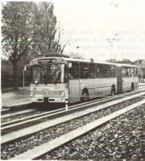
FIGURE 3 O-Bahn guideway and articulated vehicle in Essen (1).
