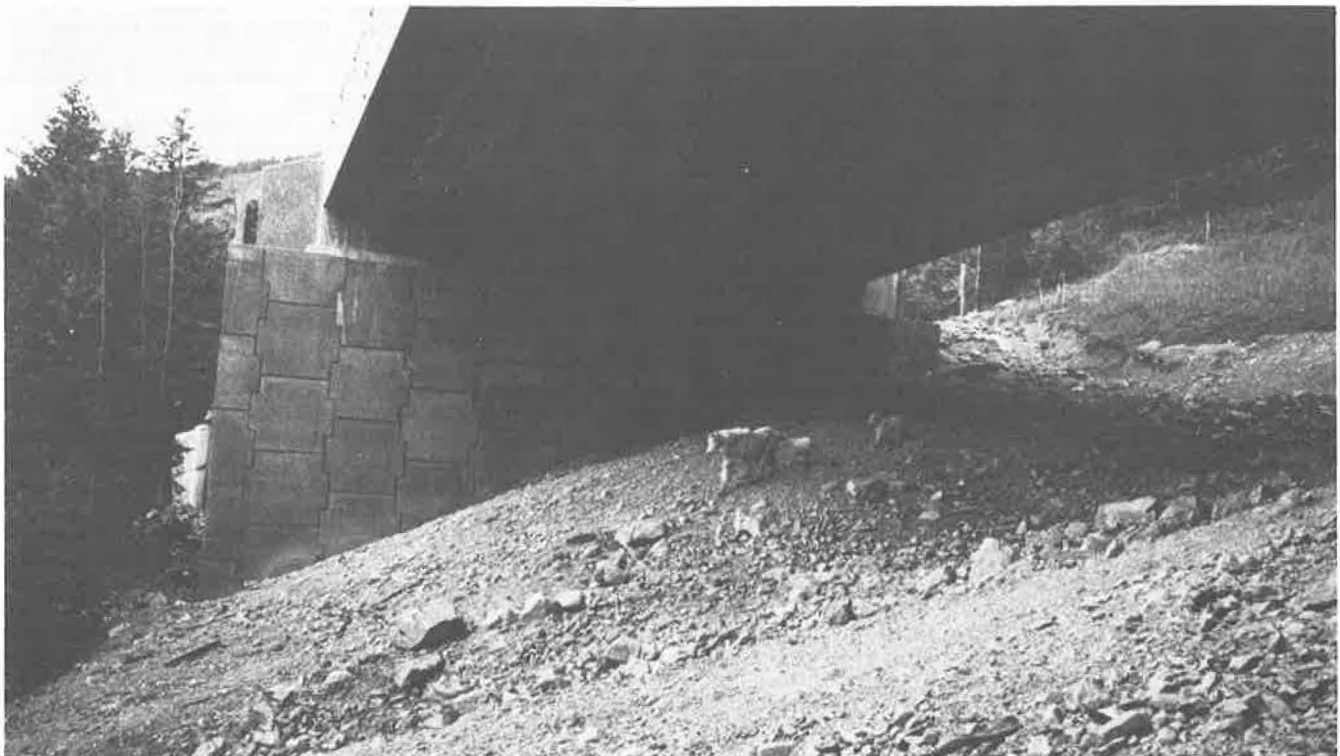
FIGURE 4 Nanny with twins at side passing under the Goat Bridge of US-2, Glacier National Park, Montana.
