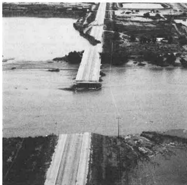
FIGURE 1 Ina Road Bridge of the Santa Cruz River in 1983—bank migration toward the foreground more than doubled the channel width.
