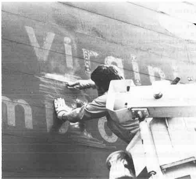
FIGURE 1 Sign preparation for System 5 material.
