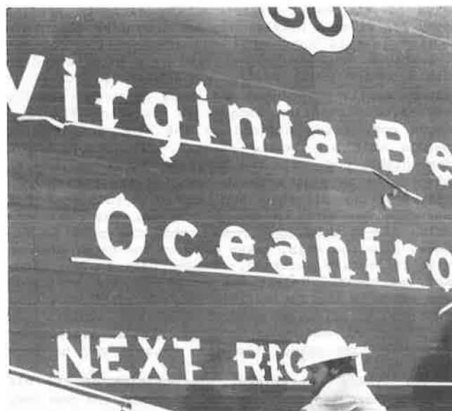
FIGURE 6 Applying copy to System 5 overlay.
