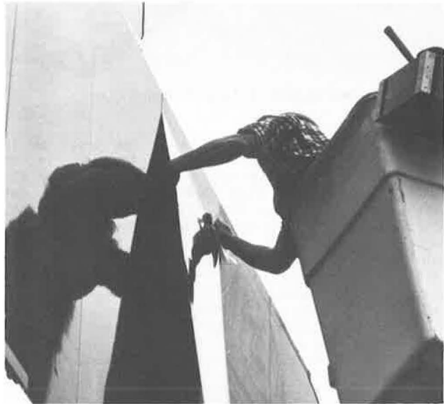
FIGURE 4 Applying System 5 sheeting.
