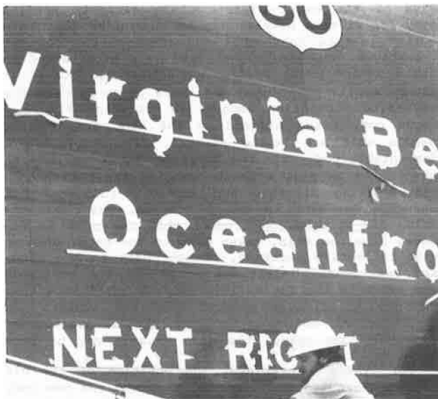
FIGURE 6 Applying copy to System 5 overlay.
