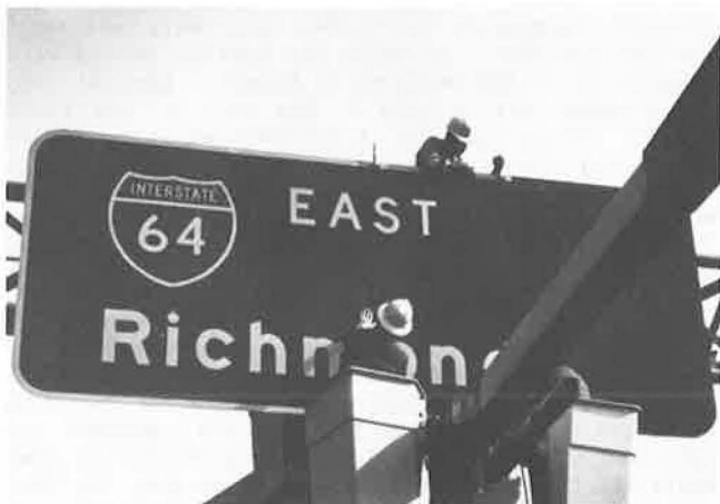
FIGURE 3 Riveting overlay panel to in-place sign.
