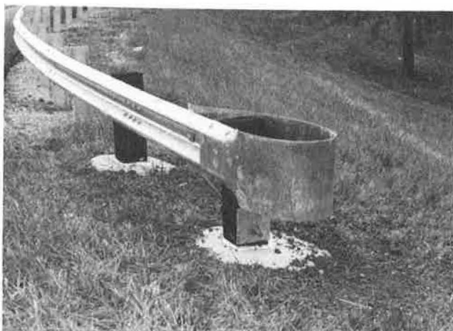
FIGURE 1 BCT end treatment (Kentucky's Type 4).
