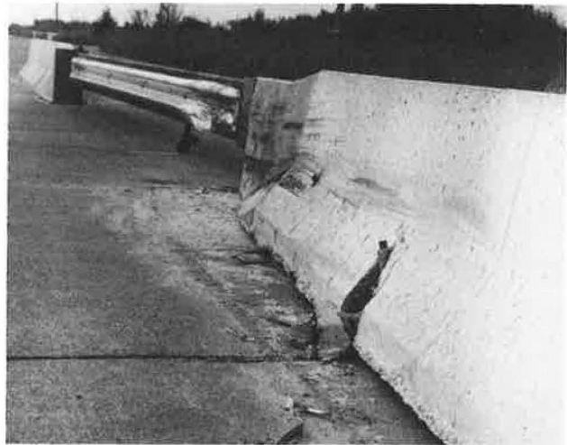
FIGURE 13 Test installation after Test 3.
