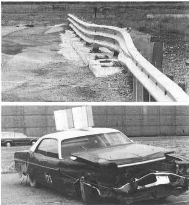
FIGURE 8 Vehicle and barrier after impact on guiderail-bridge-rail transition, Test 73.
