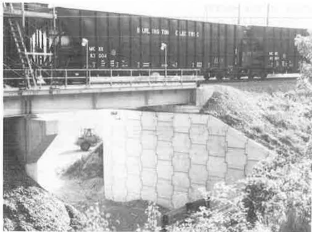
FIGURE 9 Reinforced Earth abutment at McNeil generating station.
