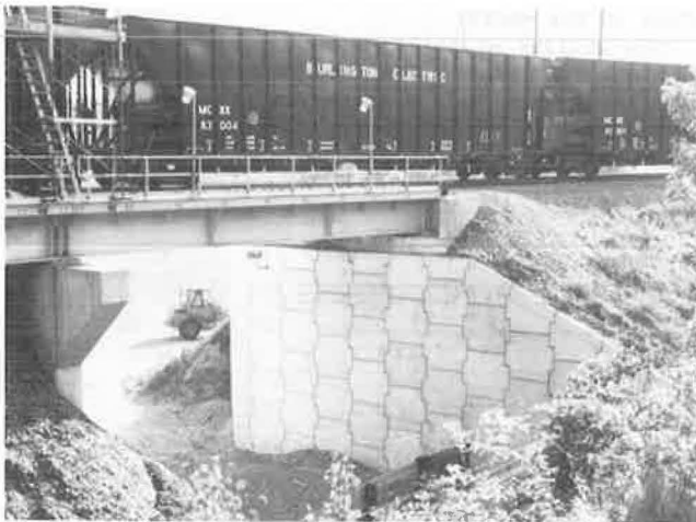
FIGURE 9 Reinforced Earth abutment at McNeil generating station.
