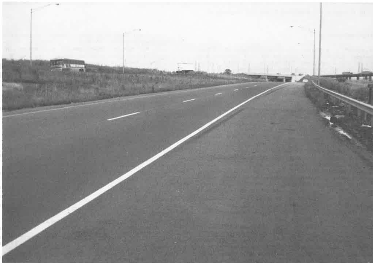
FIGURE 7 Interstate 85 eastbound, 3 years after construction.
