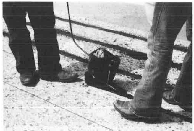
FIGURE 12 Placing PC ribbon.
