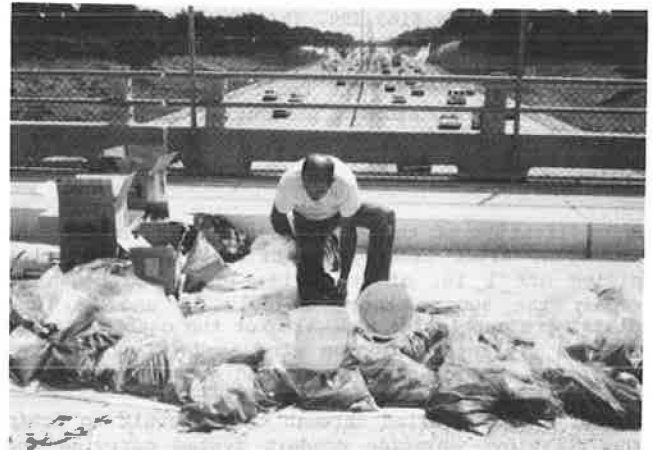
FIGURE 11 Mixing resin, hardener, and coke.
