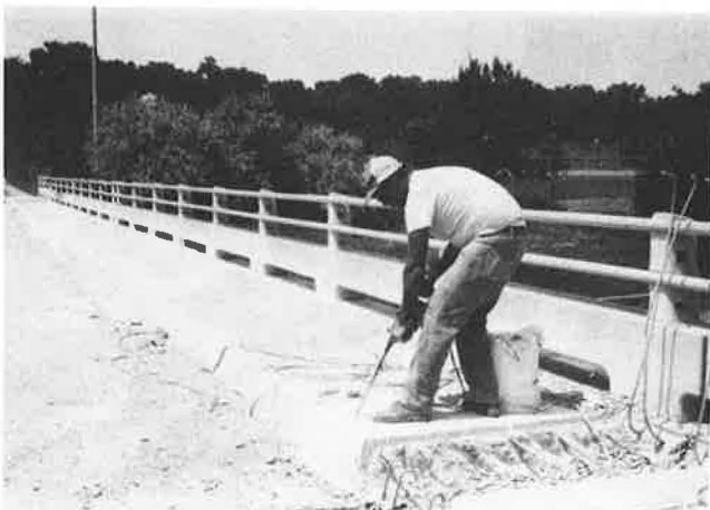
FIGURE 7 Drilling hole through curb for primary anode wire.
