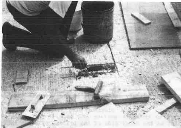
FIGURE 9 Patching reference cell.
