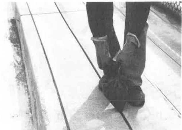
FIGURE 14 Placing conductive PC in sidewalk slot.
