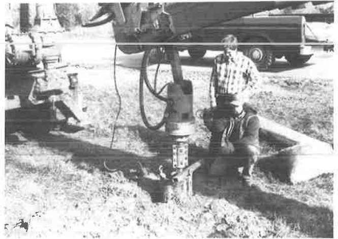
FIGURE 16 Drilling in casing.
