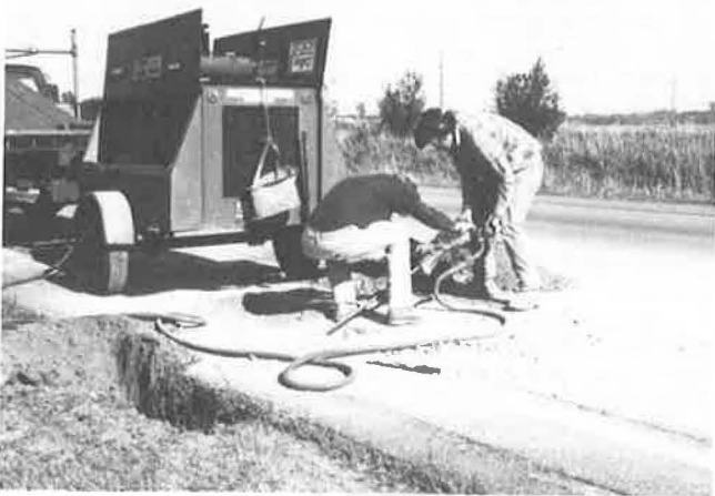
FIGURE 10 Drilling under bituminous shoulder.
