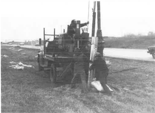
FIGURE 15 Lowering canister into post hole.
