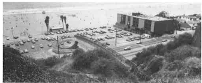
FIGURE 22 Montana Pedestrian Overcrossing.
