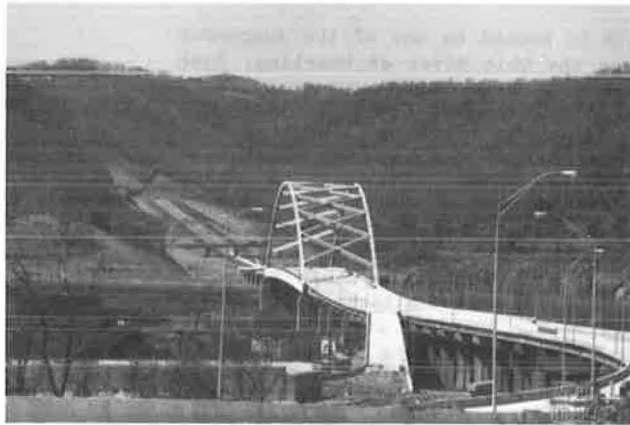
FIGURE 2 General view of bridge (looking northwest).
