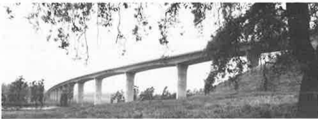
FIGURE 21 Napa River Bridge.
