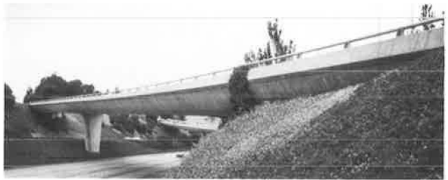
FIGURE 13 Curved Soffit girder.
