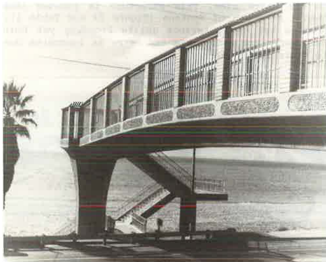
FIGURE 25 Castellamare Pedestrian Overcrossing.
