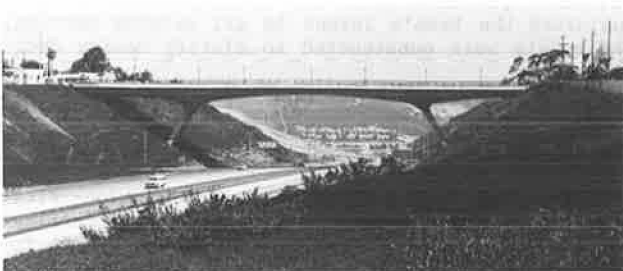
FIGURE 19 Adams Avenue Overcrossing—actual.
