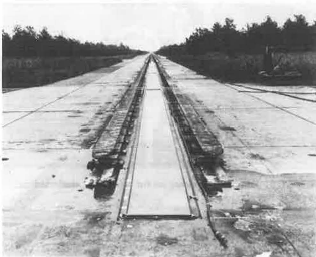
FIGURE 8 Test bed at the end of the test track.
