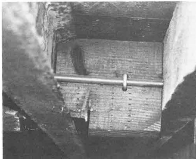
FIGURE 2 New blocking placed between existing steel and timber beams.
