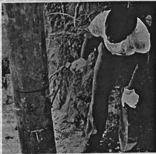
FIGURE 6 Spiral steel rod being placed at joint.
