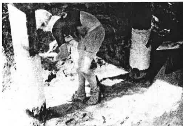
FIGURE 7 Sealing the region between epoxy trenches with gel.
