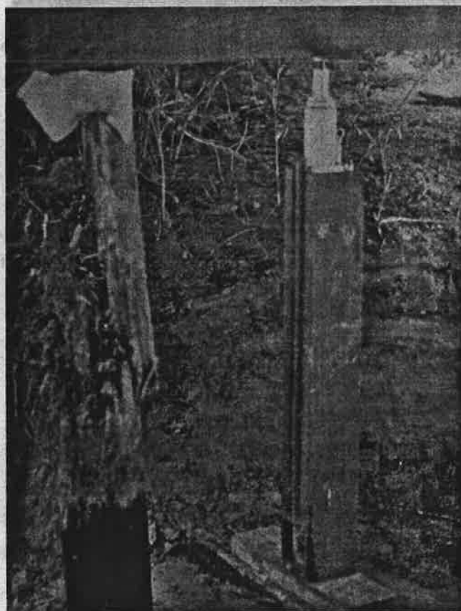
FIGURE 2 Seriously deteriorated pile with jack supporting pile cap.
