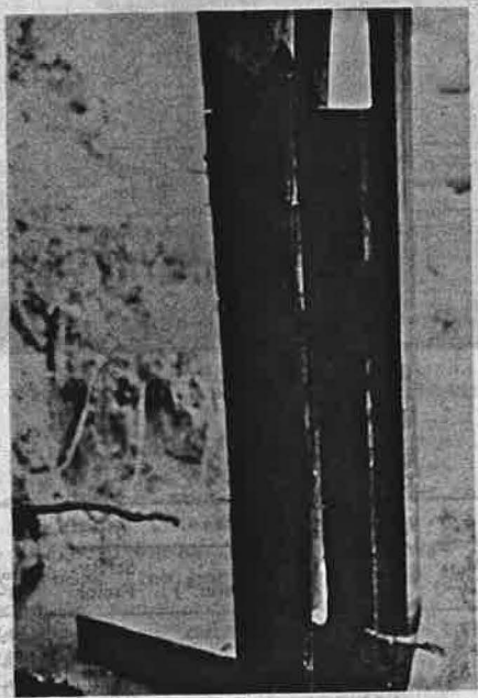
FIGURE 5 Pile with replacement section in place.
