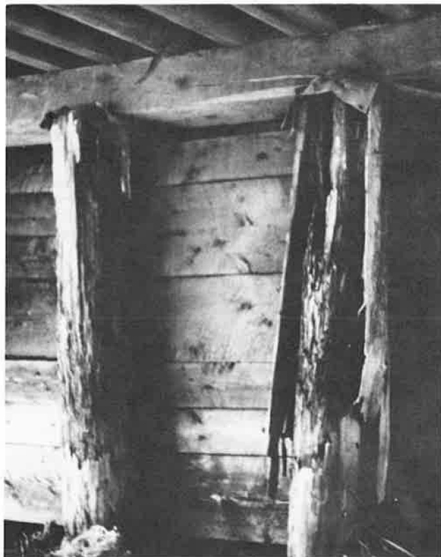
FIGURE 4 Sheet metal caps between pile tops and stringer support caps may increase decay hazard.
