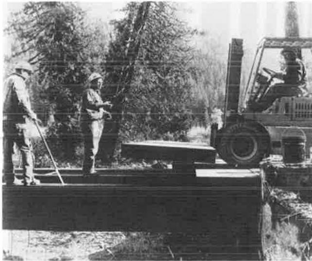
FIGURE 6 Glued-laminated deck slabs being installed as a replacement deck on a 12-year-old bridge.
