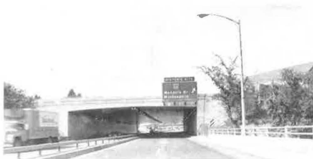
FIGURE 2 Test tunnel, view 1.
