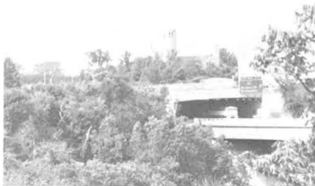
FIGURE 3 Test tunnel, view 2.
