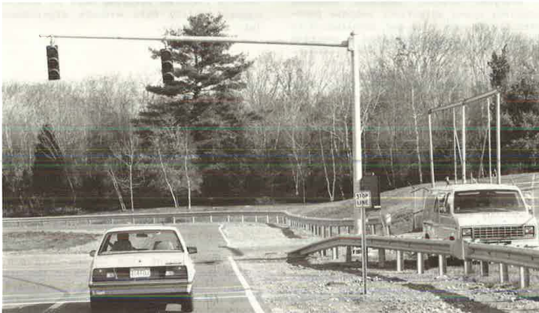
FIGURE 2 Signalized intersection and instrumentation van.
