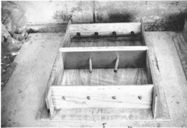
FIGURE 7 Two-dowel test: form ready for casting.
