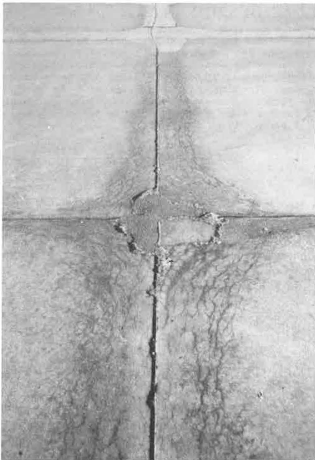
FIGURE 1 Severely D-cracked PCC pavement.
