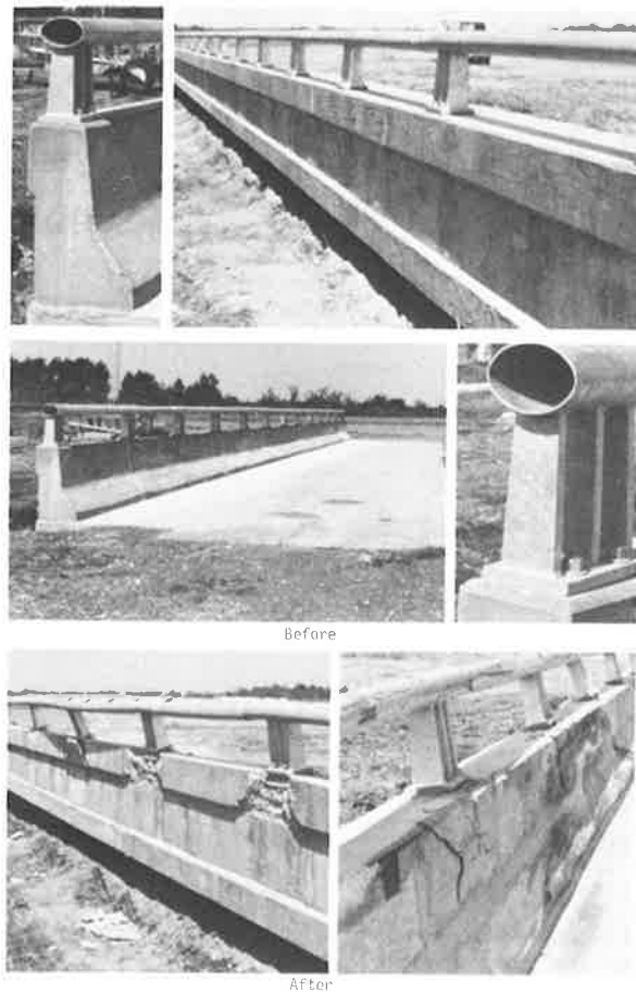
FIGURE 8 Bridge rail before and after test.
