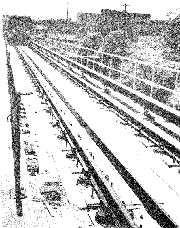
FIGURE 4 Low spring-rate, direct-fixation track on WMATA in Washington, D.C.
