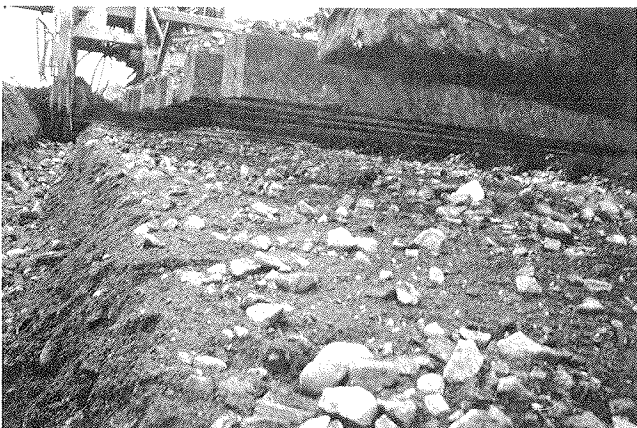
FIGURE 9 Typical condition of undercut surface prepared to receive geotextile.
