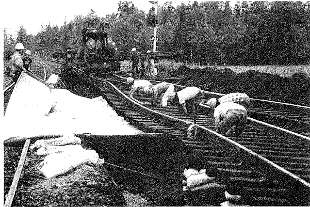
FIGURE 13 Placement of doubled-over geotextile below half area of turnout.
