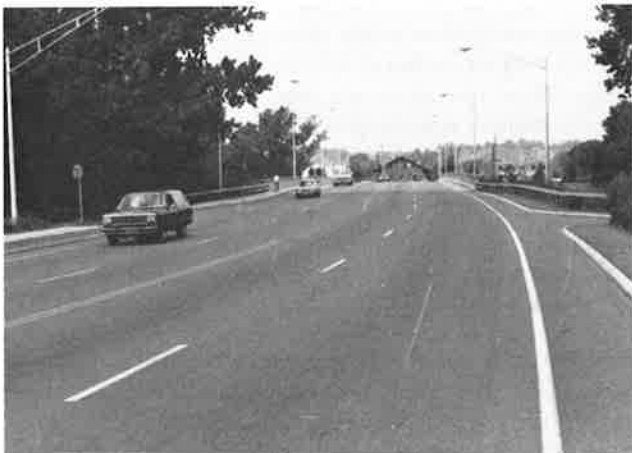
FIGURE 2 Typical epoxy markings in good condition.
