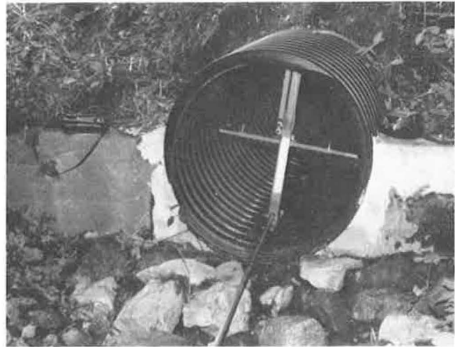
FIGURE 5 Direct-reading deflectometer for measuring deflection in 24-in. culverts.
