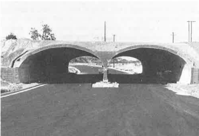
FIGURE 15 Weir Canyon—completed multiple super span.
