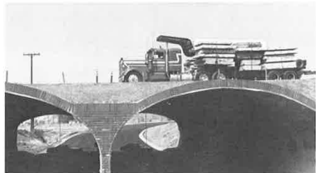
FIGURE 17 Weir Canyon—P-13 loading.
