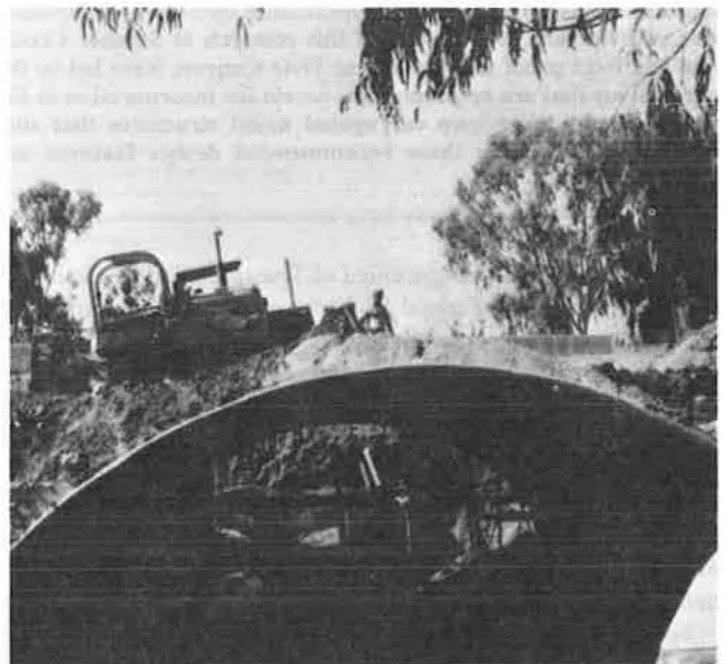
FIGURE 4 Stenner Creek—compacting structure backfill.
