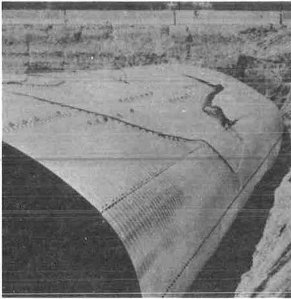
FIGURE 1 Stenner Creek—structural plate assembly.
