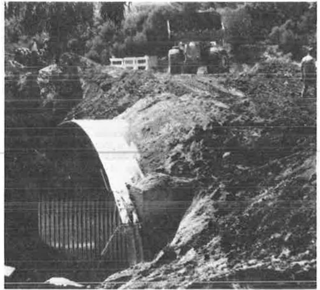
FIGURE 3 Stenner Creek—backfilling.
