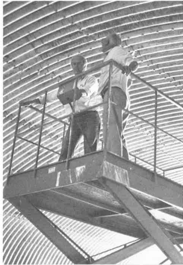
FIGURE 16 Weir Canyon—monitoring deflection.
