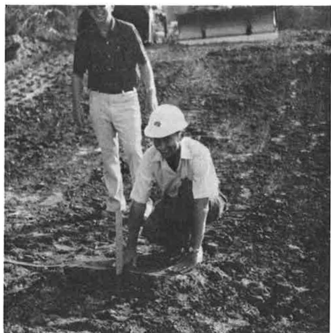
FIGURE 8 Stenner Creek—placing tape switches.
