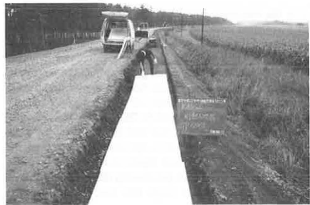
FIGURE 4 Placement of insulation boards in road shoulder.
