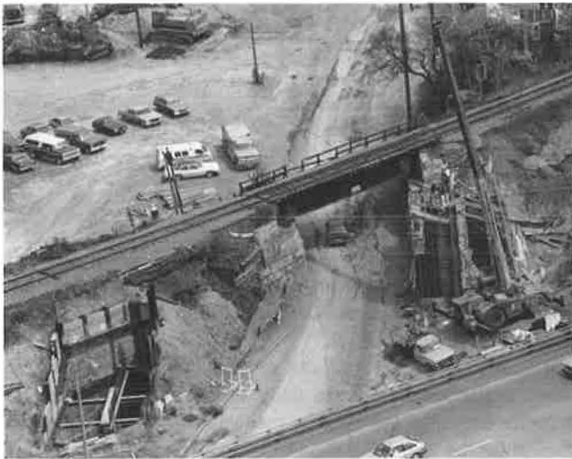
FIGURE 1 Brighton Avenue railroad bridge under construction.
