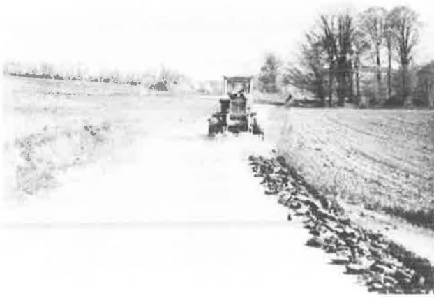
FIGURE 1 Grader scarifying roadway.
