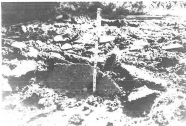
FIGURE 2 Asphalt chunks of pavement after scarifying.
