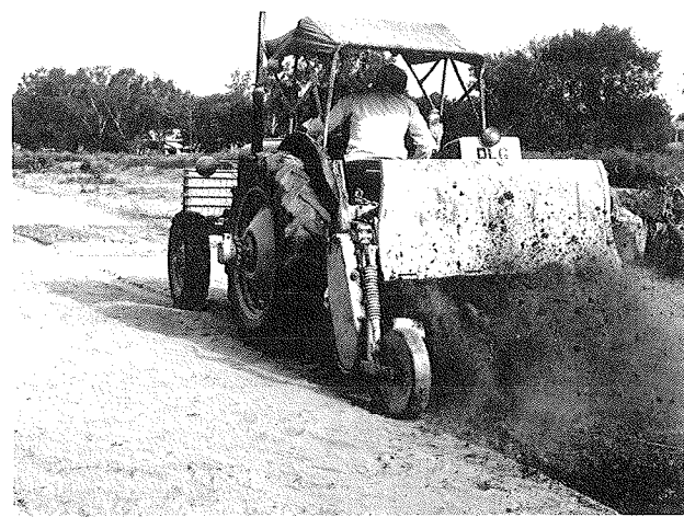
FIGURE 24 Tractor-towed Rotiller for mixing soil with stabilizer.
