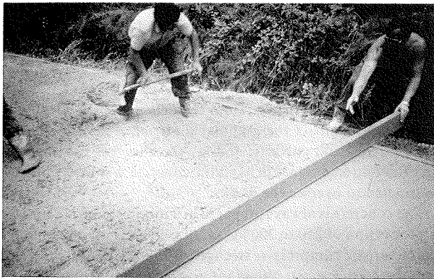
FIGURE 3 Compaction of concrete.
