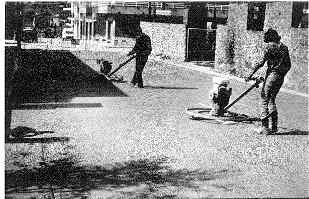
FIGURE 8 Texturing with power trowels.
