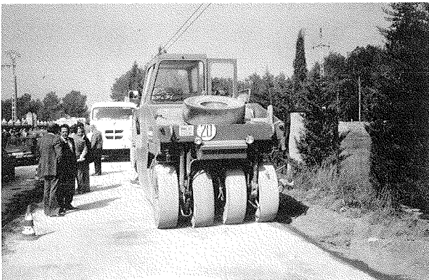
FIGURE 7 Compaction with rubber-tired roller.
