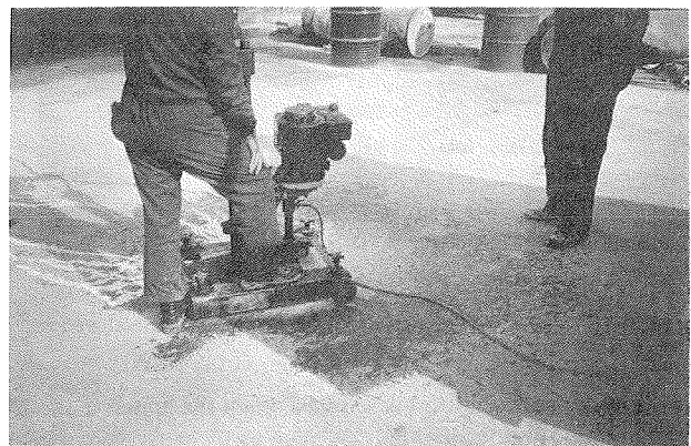
FIGURE 13 Extraction of cores.
