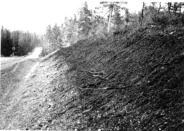
FIGURE 1 Muskeg with three tree root layers exposed in road cut.
