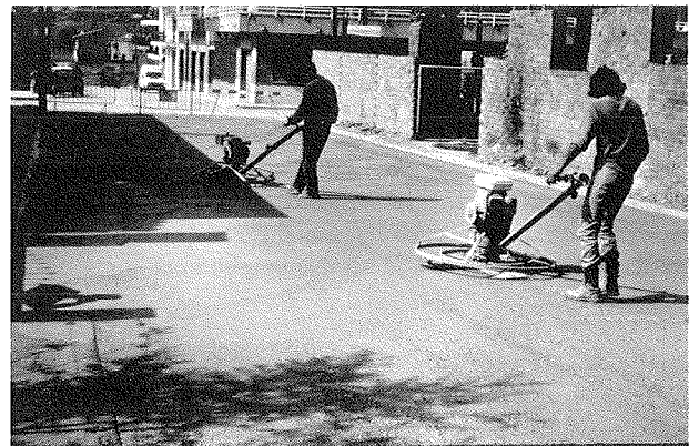
FIGURE 8 Texturing with power trowels.
