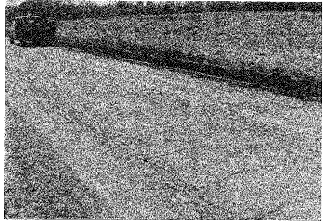
FIGURE 14 Existing road surface on the Luzerne County project.
