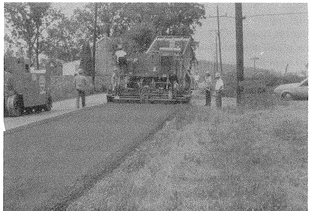
FIGURE 5 Laydown behind the Motopaver on the Chester County project.
