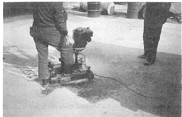
FIGURE 13 Extraction of cores.
