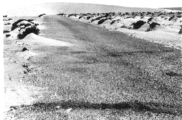
FIGURE 1 A migrating barchan has cut off the road from Laayoune to Bojador, 31.5 km from Laayoune.
