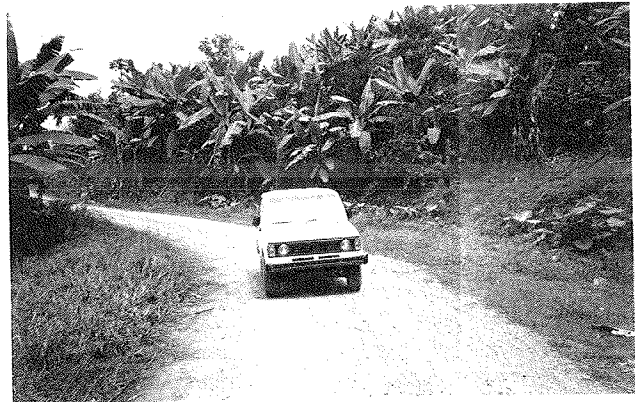
FIGURE 1 Typical 4.0 meters of gravel road.
