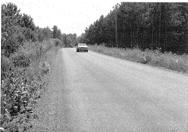
FIGURE 13 Roadway after double surface treatment on the Susquehanna County project.
