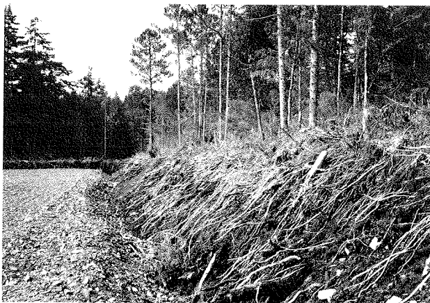
FIGURE 2 Tree roots exposed throughout muskeg excavation.
