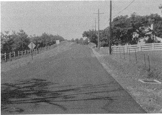
FIGURE 6 Completed roadway on the Chester County project.
