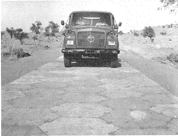
FIGURE 21 A demonstration stretch in which a special pavement system was adopted for sandy areas.
