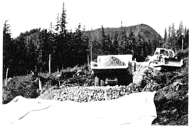
FIGURE 4 Placing 8-in minus rock embankment on geotextile fabric.
