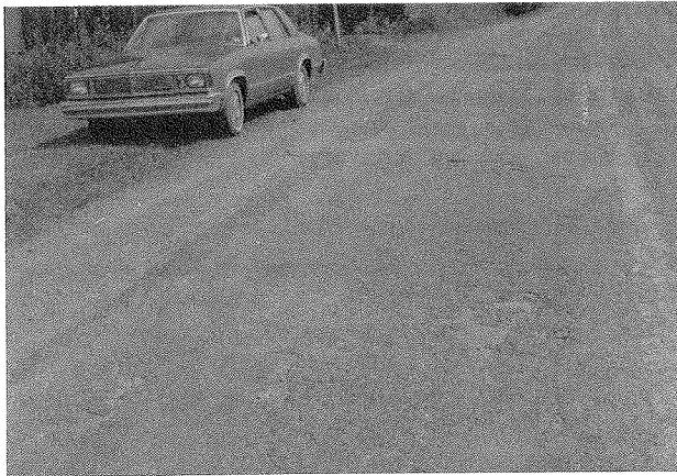
FIGURE 7 Existing road surface on the Susquehanna County project.
