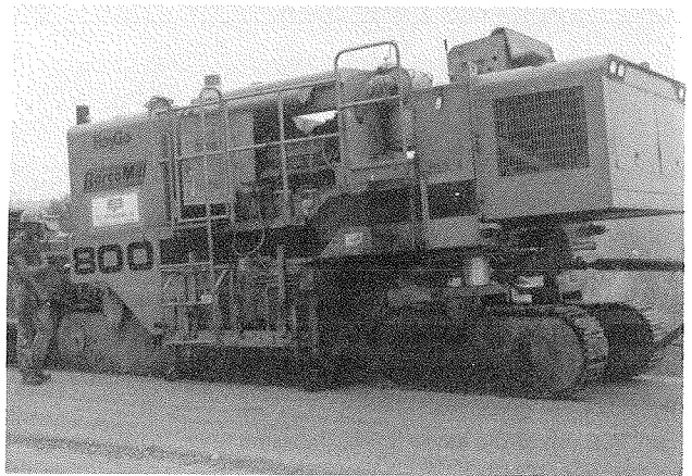
FIGURE 15 RayGo BarcoMill equipment on the Luzerne County project.
