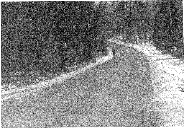
FIGURE 17 Roadway after the first winter on the Luzerne County project.
