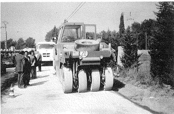
FIGURE 7 Compaction with rubber-tired roller.
