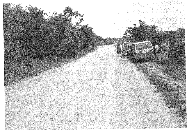
FIGURE 2 Typical 6.0 meters of gravel road.
