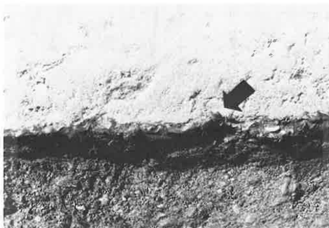
FIGURE 4 Seam of bituminous underseal exposed during installation of edge drain.
