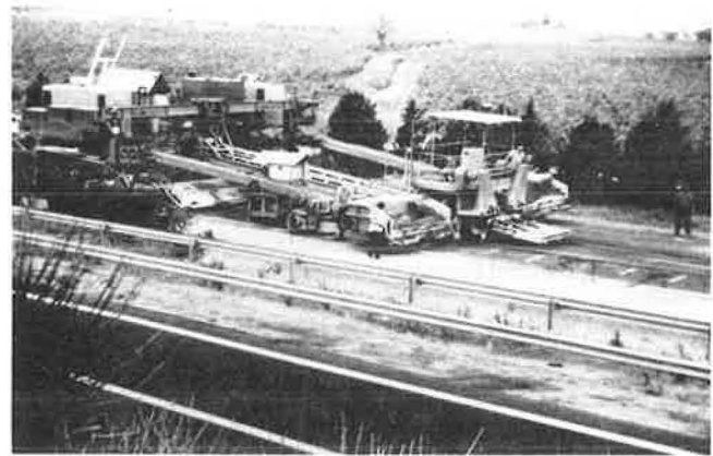
FIGURE 1 A compact paving spread.
