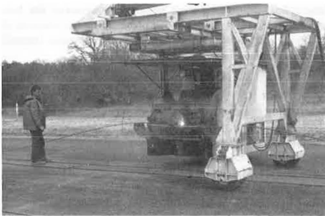
FIGURE 4 A machine flash-butts the longitudinal re-bars.
