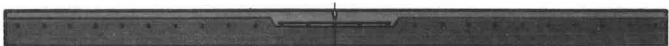
FIGURE 5 A transverse section of the double layer monolithic continuously reinforced concrete pavement used on the A71 motorway.
