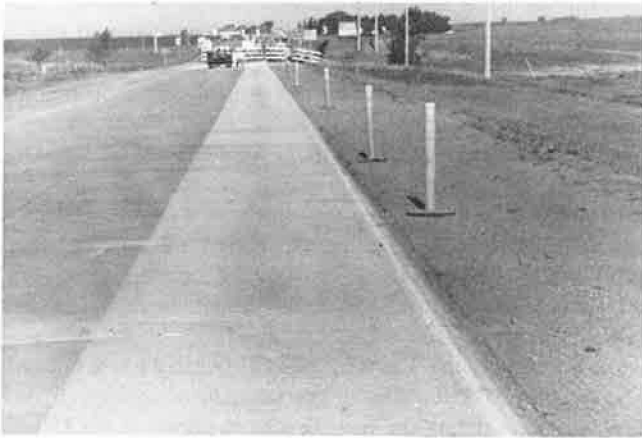
FIGURE 5 Clean concrete after one shotblaster pass.
