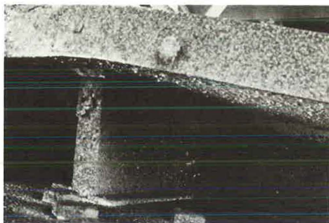
FIGURE 6 Rusty surfaces on bottom of Dollut Canal bridge before sandblasting.
