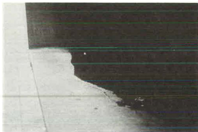
FIGURE 15 Standing water on flat floor of the statue shown in Figure 14.
