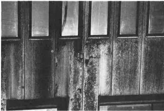
FIGURE 8 Weathering steel wall panel that corroded from the inside out.
