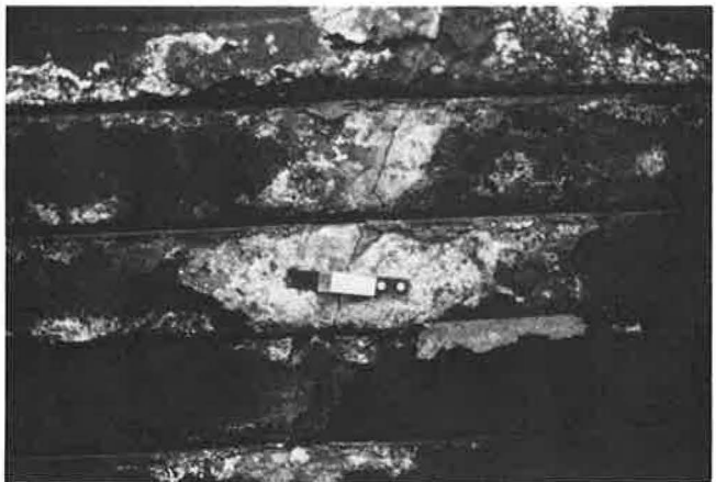
FIGURE 12 Corrosion of permanent-form decking underneath the floor slab of a parking garage.
