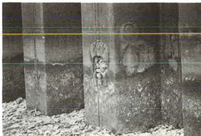
FIGURE 16 Corroded sheet piling along a tidal creek in Annapolis, Maryland.
