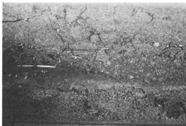
FIGURE 3 Laminar corrosion on poorly drained horizontal surface of New Jersey Turnpike highway separation bridge.
