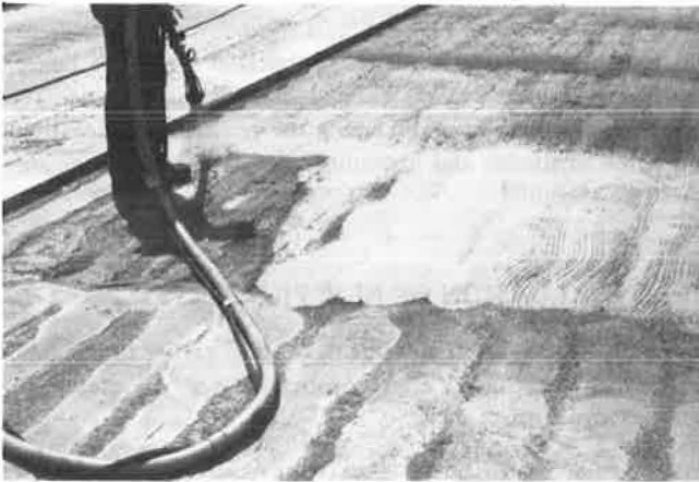
FIGURE 22 Application of Matcor/Thoro conductive coating.
