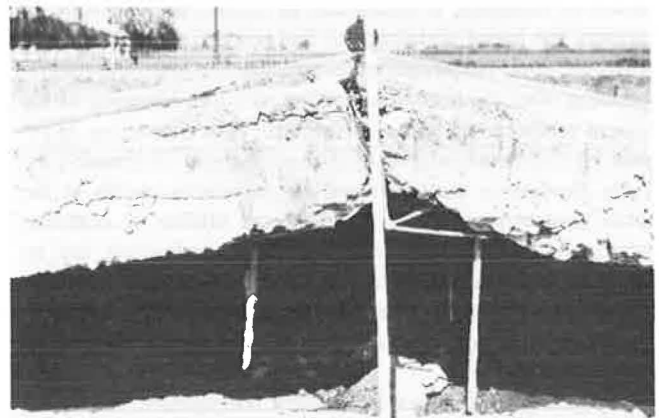
FIGURE 3 Pavement blowup.
