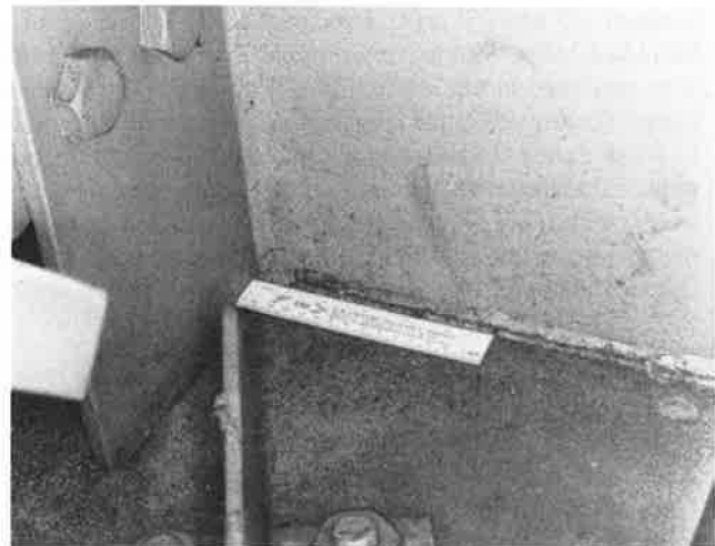
FIGURE 15 I-79 Bridge 2682 lateral gusset plate connection detail.
