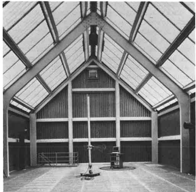
FIGURE 1 Interior of building made entirely of glass-fiber-reinforced composites.
