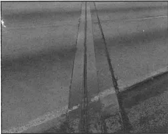
FIGURE 7 A typical neoprene compression seal dam.
