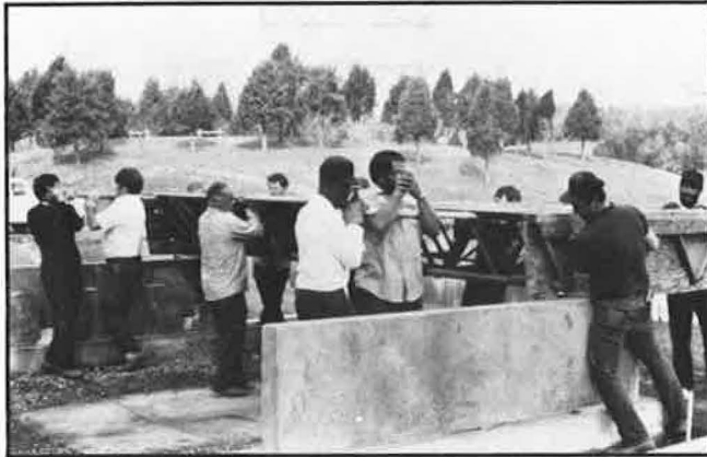
FIGURE 3 Lifting superstructure onto the precast concrete seats.
