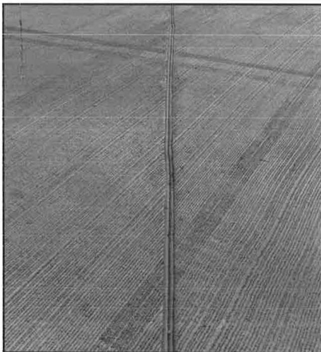
FIGURE 10 Preformed neoprene is twisted—probably a construction defect.
