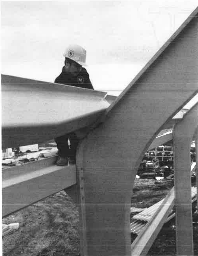
FIGURE 5 Deep rigid-frame knee without splice or connections reduces stress levels and eliminates problem of fasteners at high-moment corner.
