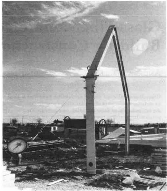
FIGURE 3 This rigid frame is being tested with an 8,000-lb lateral load at the eave to check for stiffness of the frame and fixity of the base. Box section yields good stiffness in both planes, therefore, lateral support is not needed (a real advantage in erecting operations).
