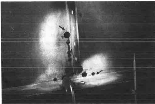
FIGURE 9 Retrofitting distortion-induced web cracking.
