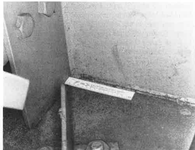
FIGURE 15 I-79 Bridge 2682 lateral gusset plate connection detail.
