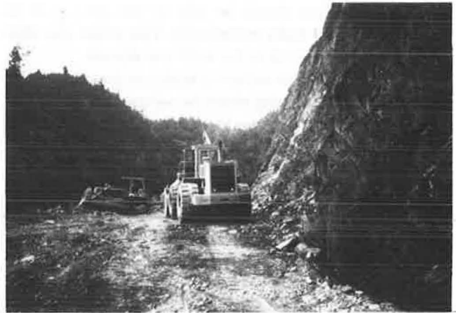
FIGURE 7 Removing broken rock from track.
