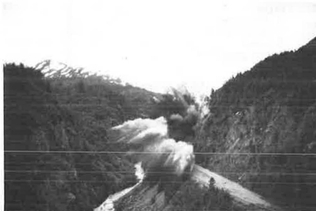
FIGURE 6 Blast detonation initiated above north portal.
