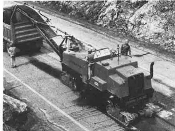
FIGURE 2 Cold milling equipment.
